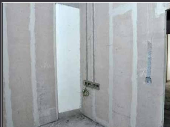
Electrical Conduit work on 75mm thick Vpanels
